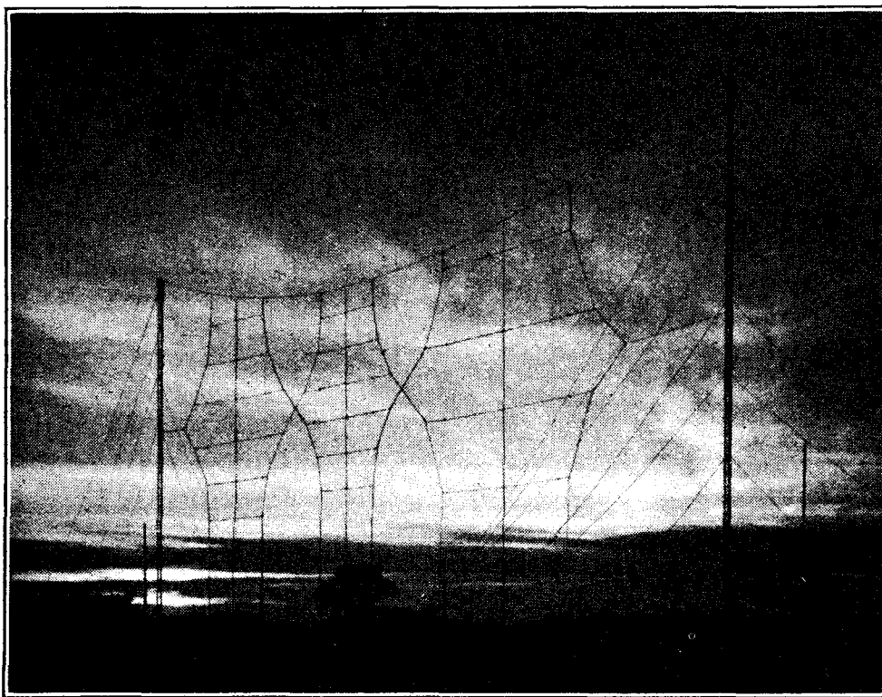
The B.B.C. engineers are well ahead of all others in the development of short-wave broadcasting. Nor do they seem disposed to rest on their laurels. Above is a sunset view of one of the Empire "arrays" at Daventry.
