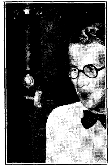
HENRY HALL is still unperturbed by the demolition work on Waterloo Bridge, next to "No. 10" studio.
